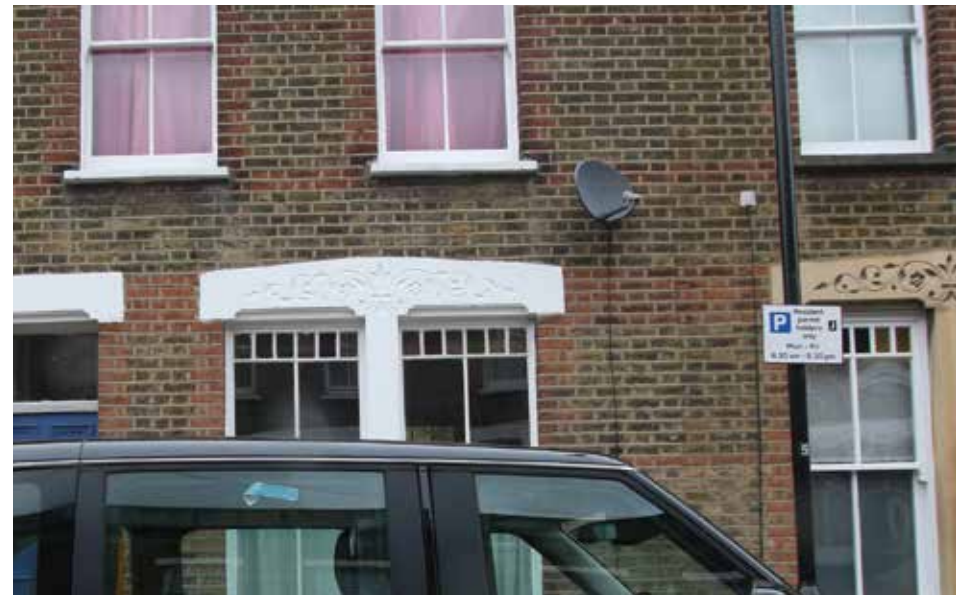
Satellite dishes detract from the conservation area
