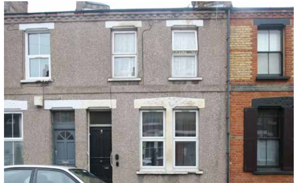
Innapropriate pebble dash render obscuring historic detailing
