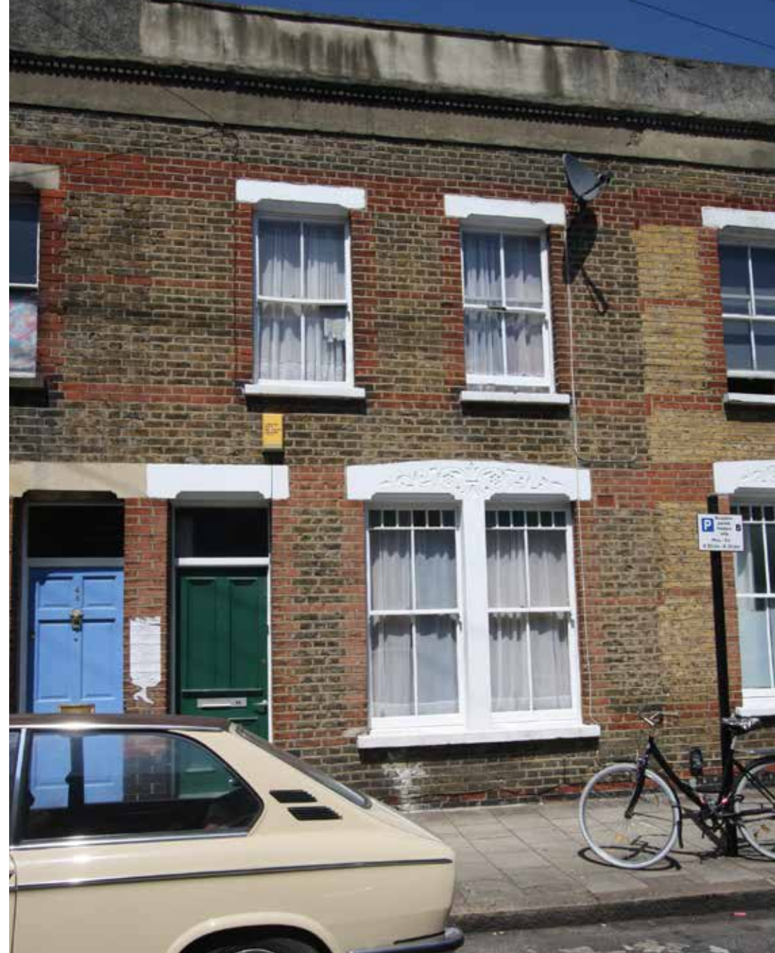
Beck Road with hidden butterfly roof behind chunky parapet
